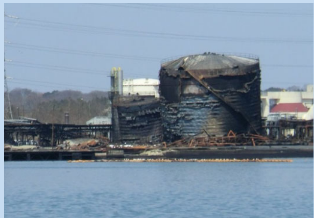
Figure 5: Burned tanks at the Sendai refinery hit by the tsunami (Photo Credit: C. Scawthorn)
