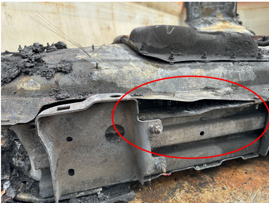
Figure 5.10 Opening on the side of the battery pack of approx. 4 cm
