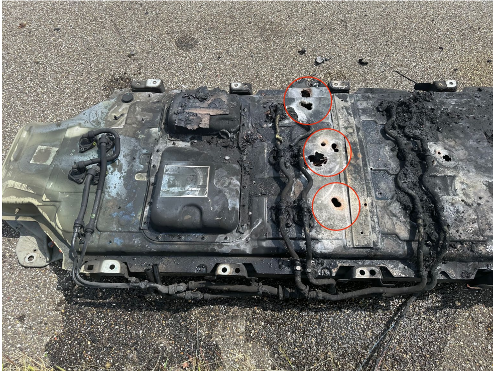
Figure 5.4 Holes cut by deployment of the UHP extinguishing system
