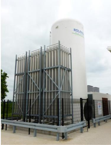
Storage tank with heat exchanger
