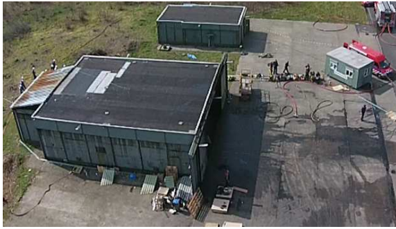
Figure B1.5 Upper view of the industrial hall
