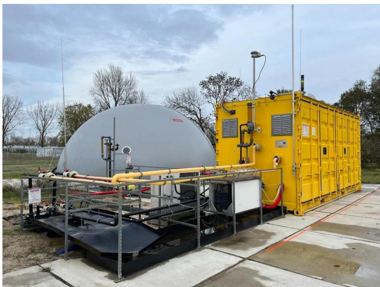
Figure 2.3 Hydrogen Bromide flow battery from Elestor (picture: Cosima Stähler)
