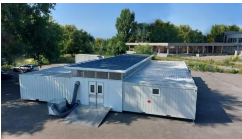
Figure 2. Field hospital built with containers.
