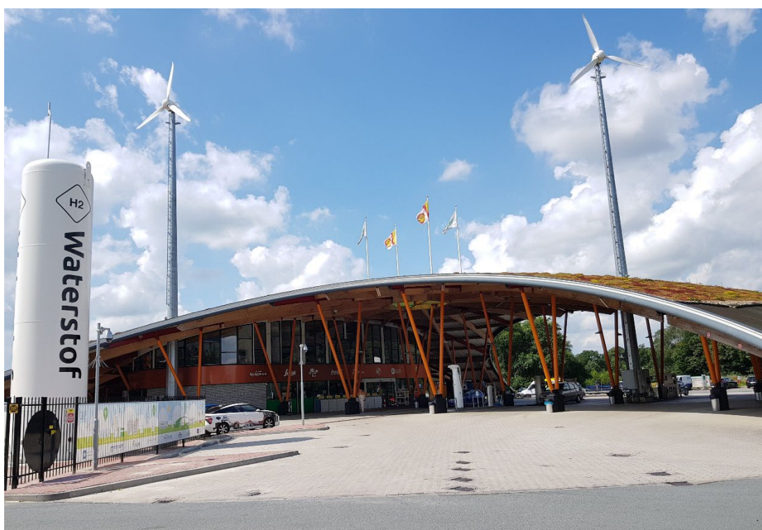
Figuur 2.1 Multi-energie station Pesse (Foto: NIPV)
