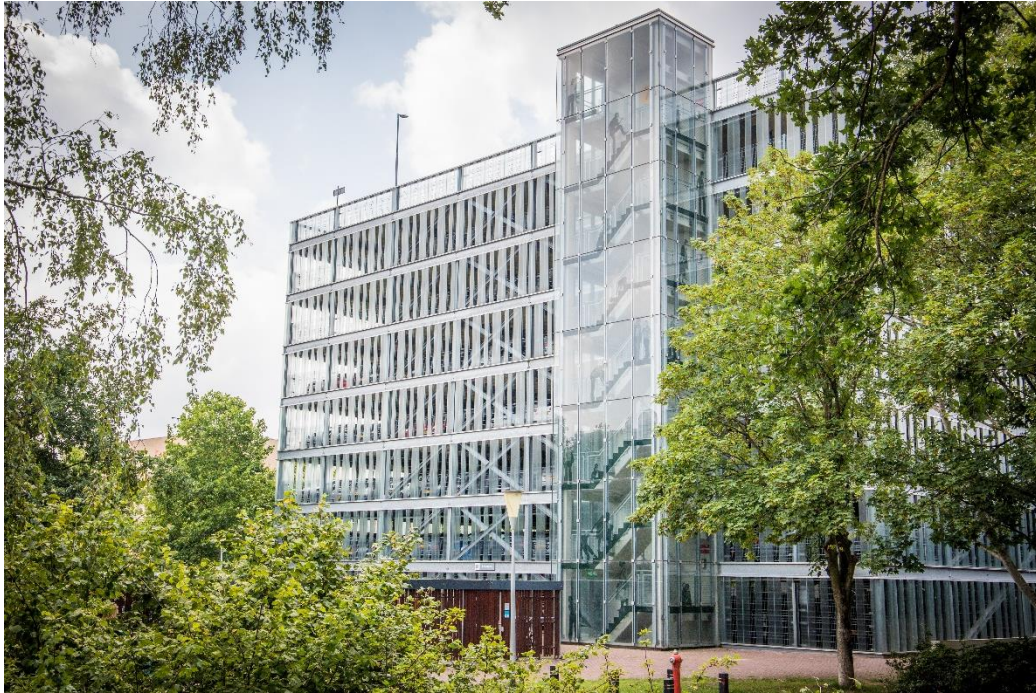
Figure 5.1 Open indoor car park (source: Tom Hessels, NIPV)
