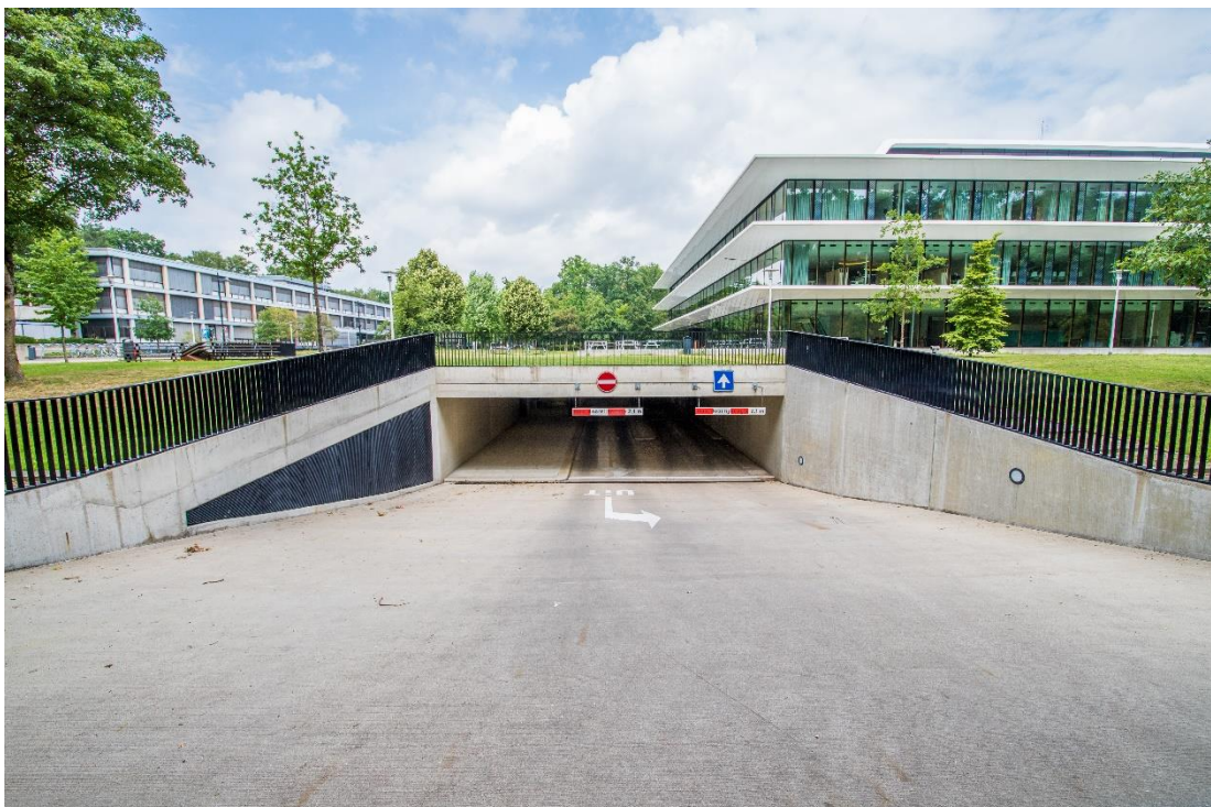
Figure 5.4 Underground car park (source: Tom Hessels, NIPV)
