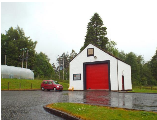
Figuur 5.1 Bridge of Orchy community fire station, Schotland (foto: © Malc McDonald (cc-by-sa/2.0))
