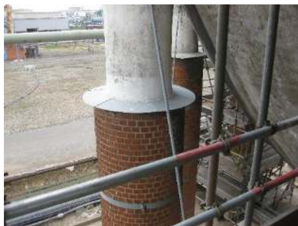
Figure 48 – Watershedding Detail to Prevent Water Ingress
