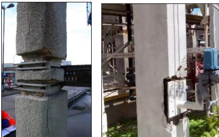
Figure 49 - Examples of removal of PFP to add attachments/penetrations
