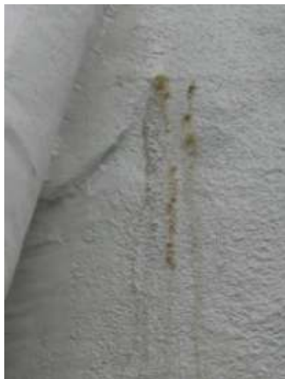
Figure 12– Salts being Washed from Epoxy PFP Material
