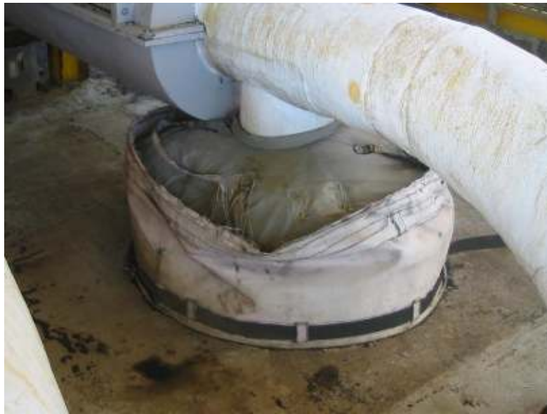
Figure 41 – Detailing PFP Interfaces (Dry-fit, Coating, Jacket)
