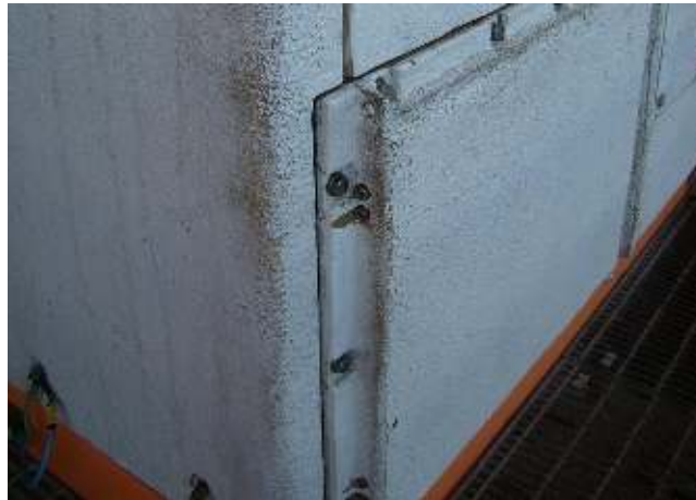
Figure 23 - Epoxy intumescent dry-fit construction with sealed joints
