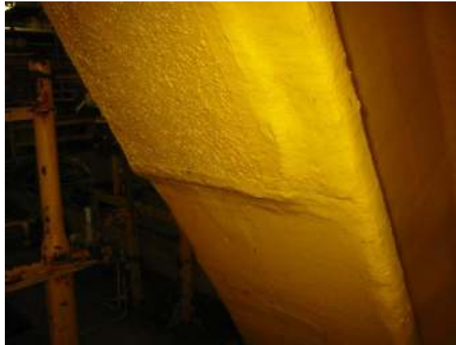
Figure 51 – Repair of LWC material with an epoxy intumescent.
