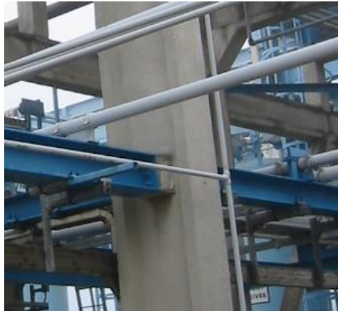
Figure 46 - Structural steelwork without coatback
